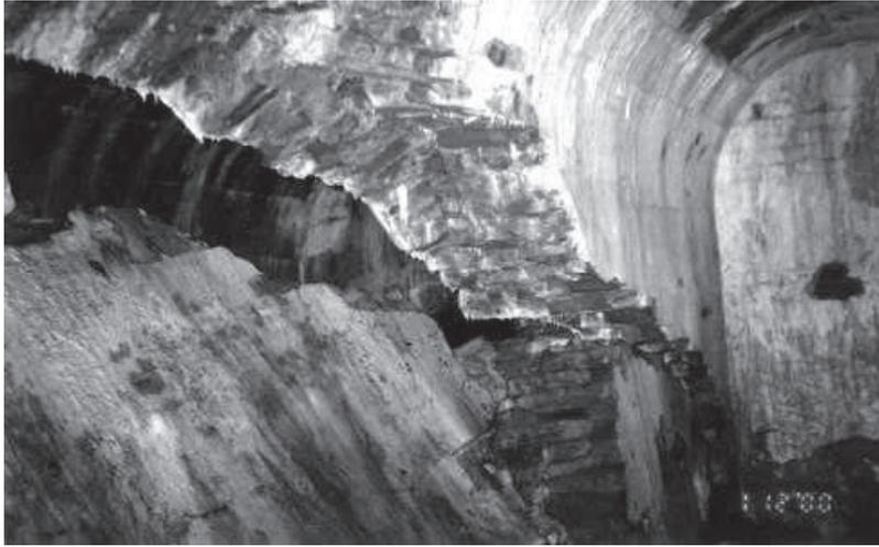
Figure 18. Collapsing cellar wall behind east loggias.
