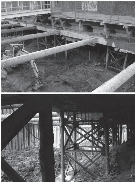
Figure 7. Strutting tubes are installed between the top slab and the sheet pile wall. Excavation for the underground space under the theatre below and around the footprint.
