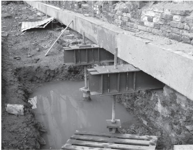
Figure 3. Introduction of beams underneath the waling and transferring loads onto piles.
