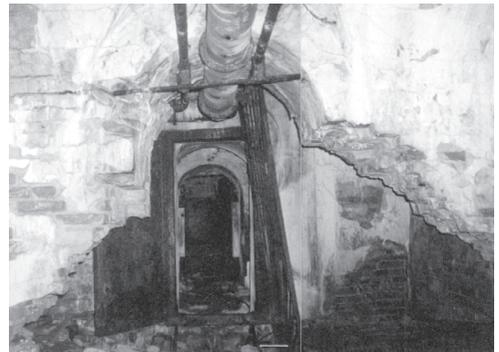
Figure 15b. Dilapidated structures of the palace: transverse walls.
