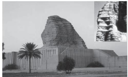
Figure 2. Ziggurat Aqar-Quf, 3500 year old reinforced soil structure near Bagdad (picture by unknown reference)
