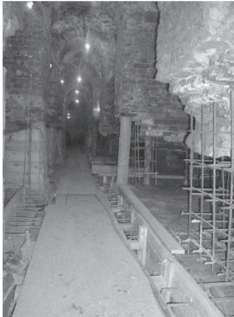
Figure 25. Deepening of the basements by 1.0-1.5 m.
