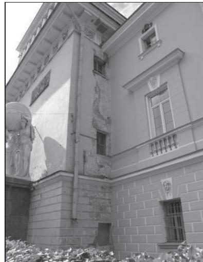
Fig. 33. Development of cracks in the Admiralty tower
