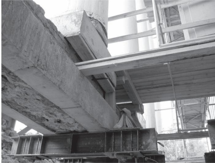
Figure 4. All loads have been redistributed. Old foundations removed.
