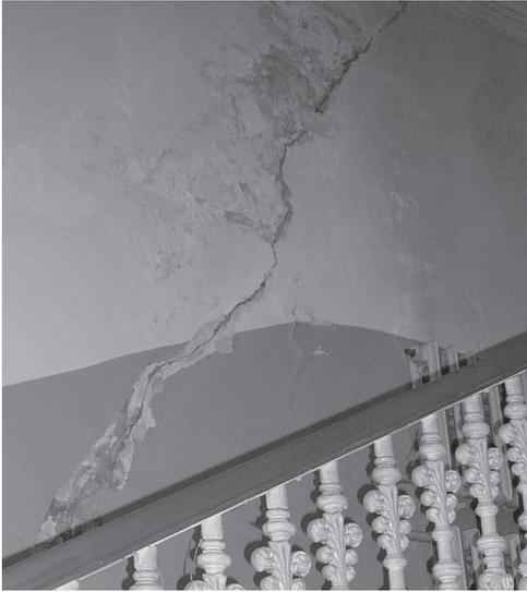
Fig. 36. Cracks in the wall of stairwell passage
