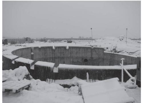
Figure 1. The reservoir after underpinning with bored piles and the tilt having reached 1200 mm
