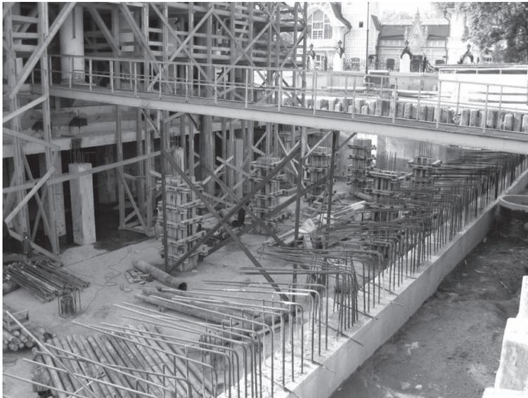
Figure 9. Constructing the underground structure.
