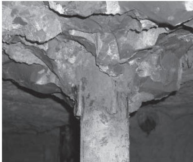
Figure 26. Bored pile with tube reinforcement viewed from underneath foundation.
