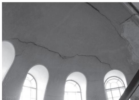
Fig. 35. Cracks in the vaults of the cathedral
